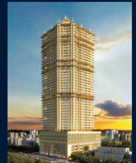
Dream Atlantis Khadakpada, Kalyan (W) 45-Storeyed Residential Landmark
