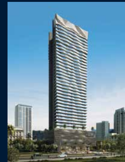
Dream Avalon Khadakpada, Kalyan (W) 34-Storeyed Residential Landmark
